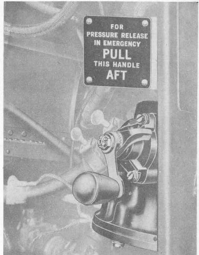
Figure 25—Main Fuel Tank Pressure Regulator
